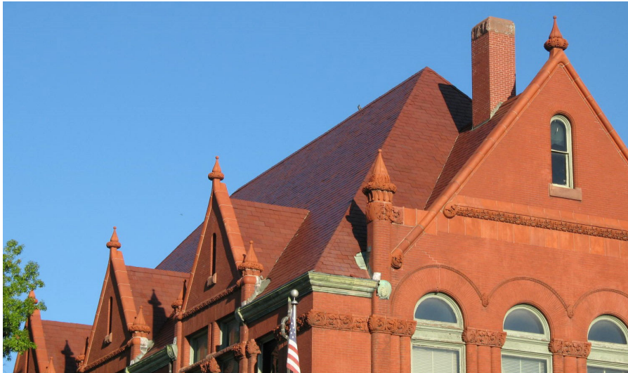
Figure 1: 120-year old New York red slate roof in Lawrence, Kansas
